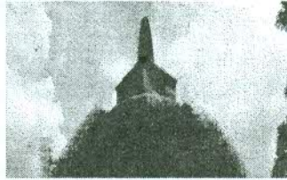
(Preservation Abayagiriya stupa)
